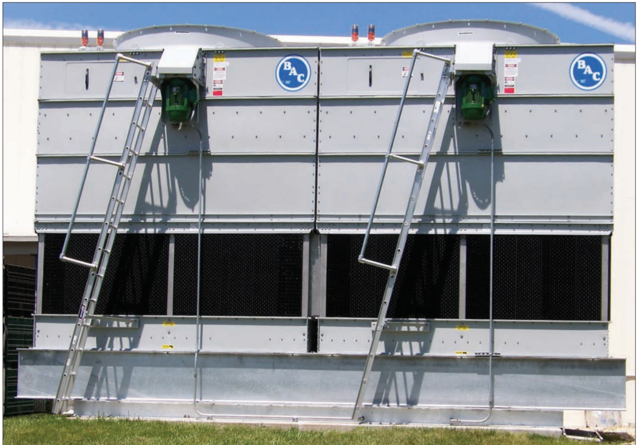
Two-cell PT2 Installation
