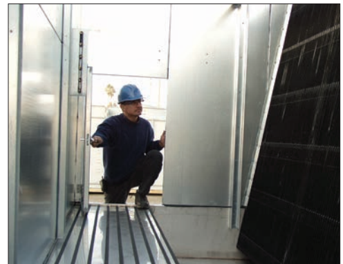
Standard Internal Walkway
