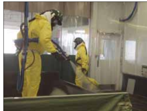
Application of TriArmor® Corrosion Protection System
