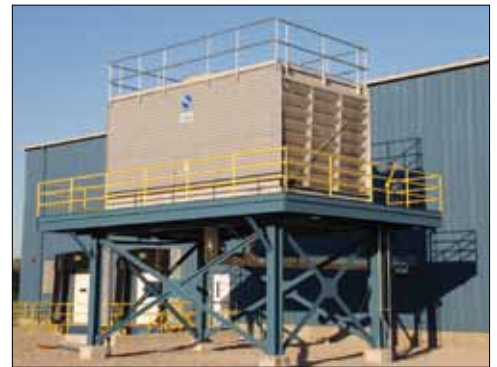
EVERTOUGH™ Construction Installation
