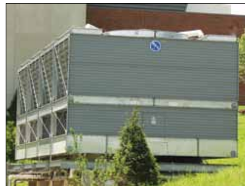
Standard Construction Installation
