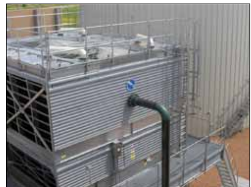
Seismic/Wind Upgraded Structure with Fiberglass Reinforced (FRP) Casing Panels
