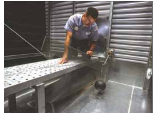
Mechanical Water Level Control
