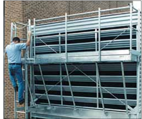
External Ladder and Platform
