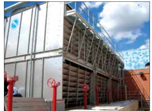
Factory Assembled Louver Face Platforms
