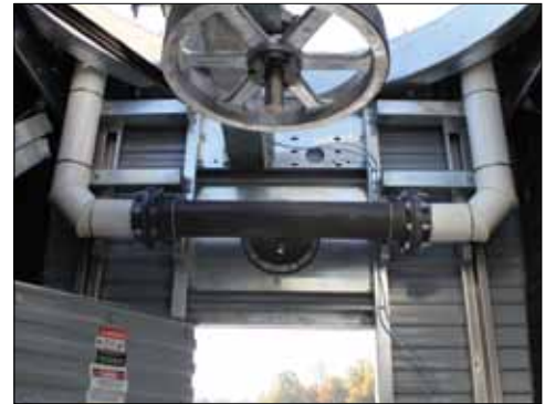
EASY CONNECT® Piping Arrangement
