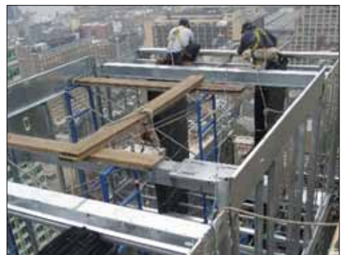
Knockdown Unit Installation
