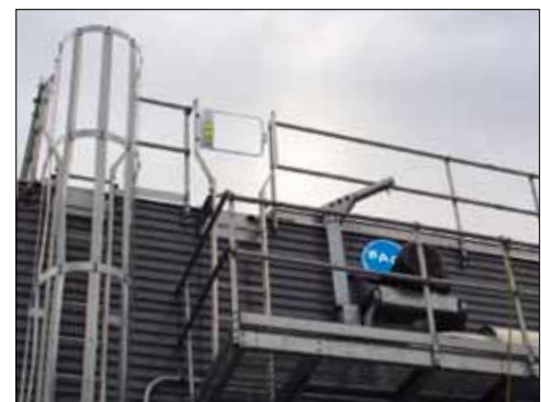
Motor Removal System with Davit Arm, Motor Access Platform, and Handrail Package
