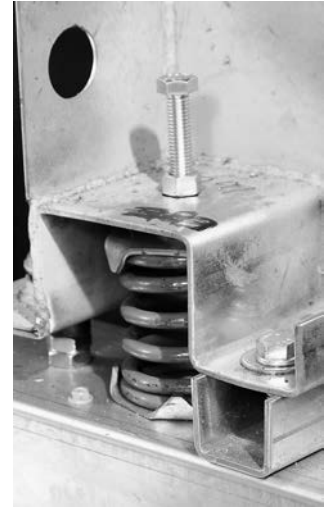
Figure 6. Spring isolation
