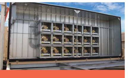
**Direct-Drive Plenum (DDP) fan arrays** allow up to 100 percent redundancy for greater systems reliability and up to 10 percent increased efficiency.
